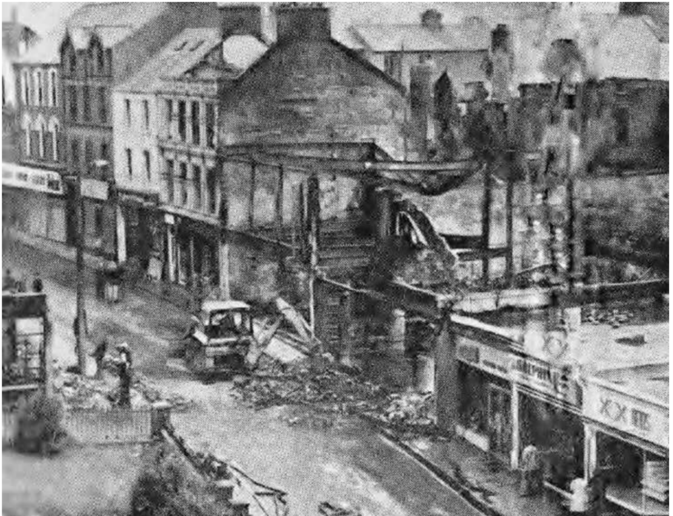
A picture of devastation. This area of Main Street, pictured on the morning after the terrorist bomb attack of 14 August 1976, suffered most damage with several shops and business premises destroyed. Other parts of the town were also attacked, causing similar damage
